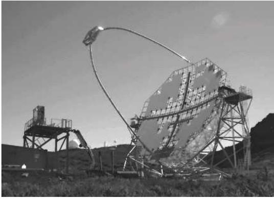
**Fig. 2** View of the MAGIC telescope in October 2002, right before the installation of the camera, visible on the access tower on the left. About 40% of the mirrors (covered at the time by protective white foils) were already in place.
