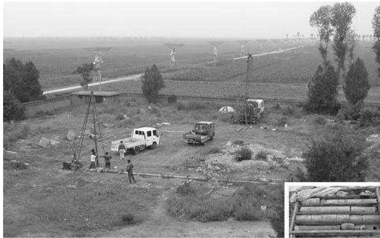
**Fig. 1** The picture shows the prospecting apparatus on the site. Some samples of the rocks underground is shown at the bottom right corner. Photo taken in 2003.
