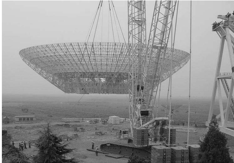
**Fig. 2** The picture shows the hoisting of the main reflector onto the pedestal. The main reflector was hoisted in one piece. Photo taken in 2005.
